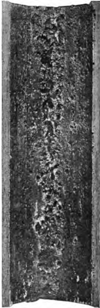
FIG. 25a.—Corroded Wrought-iron Pipe.
